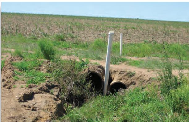
The two pipes and overfill of soil allow machinery to travel over this drainage area, not through it.
