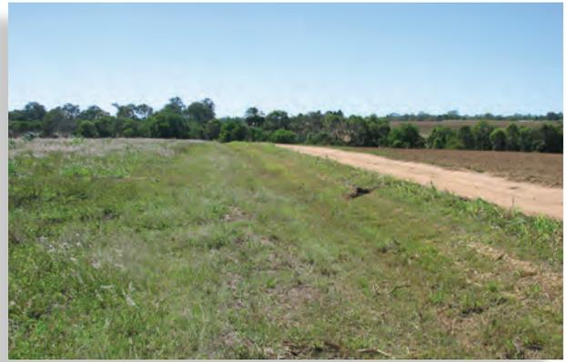
A grassed drain and diversion bank have been constructed on the uphill side of this track.
