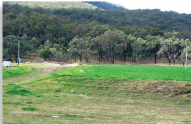
Diversion banks were established here to prevent water from the slope flowing across the paddocks and carrying topsoil into creeks and rivers. The grower maintains grassed headlands and drainage areas to divert storm water safely from the farm.
