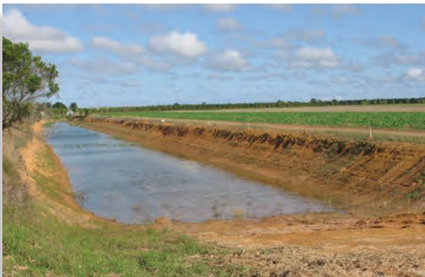
This dam collects runoff water from the vegetable farm on the right. It also acts as a silt trap. The grower can collect trapped silt from the dam when it's empty and return it to his paddocks.
