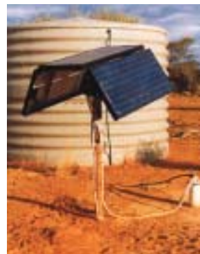
Solar powered water pump.
