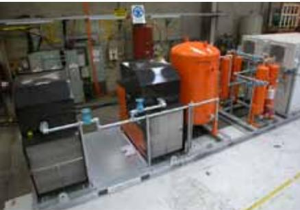
*Compressor system consisting of (left to right) a nitrogen generator used for food packaging, four air filters, a receiver tank and two compressors.*
