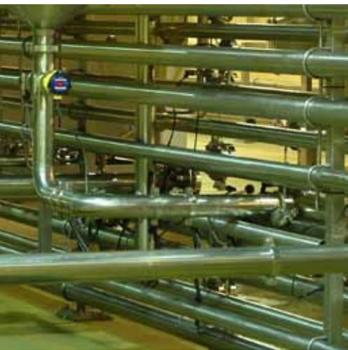
*Minimising pipework with fewer bends and dead ends will reduce cleaning requirements.*
