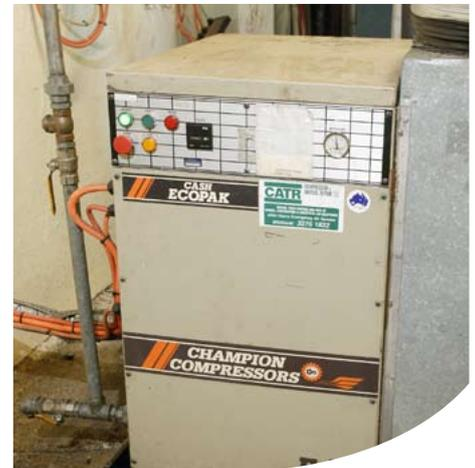
Compressed air is widely used throughout industry, accounting for about 10 percent of industrial electricity consumption and making it one of the most expensive industrial utilities. Regularly checking air compressors can reduce electricity consumption and avoid costly decreases in compression capacity.
